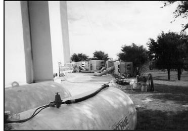
DH Tech can use different sources for power including electric, gas (propane or natural) and steam in order to run the dehumidifier in a more economical way for the customer. Here, propane is used as a power source.
